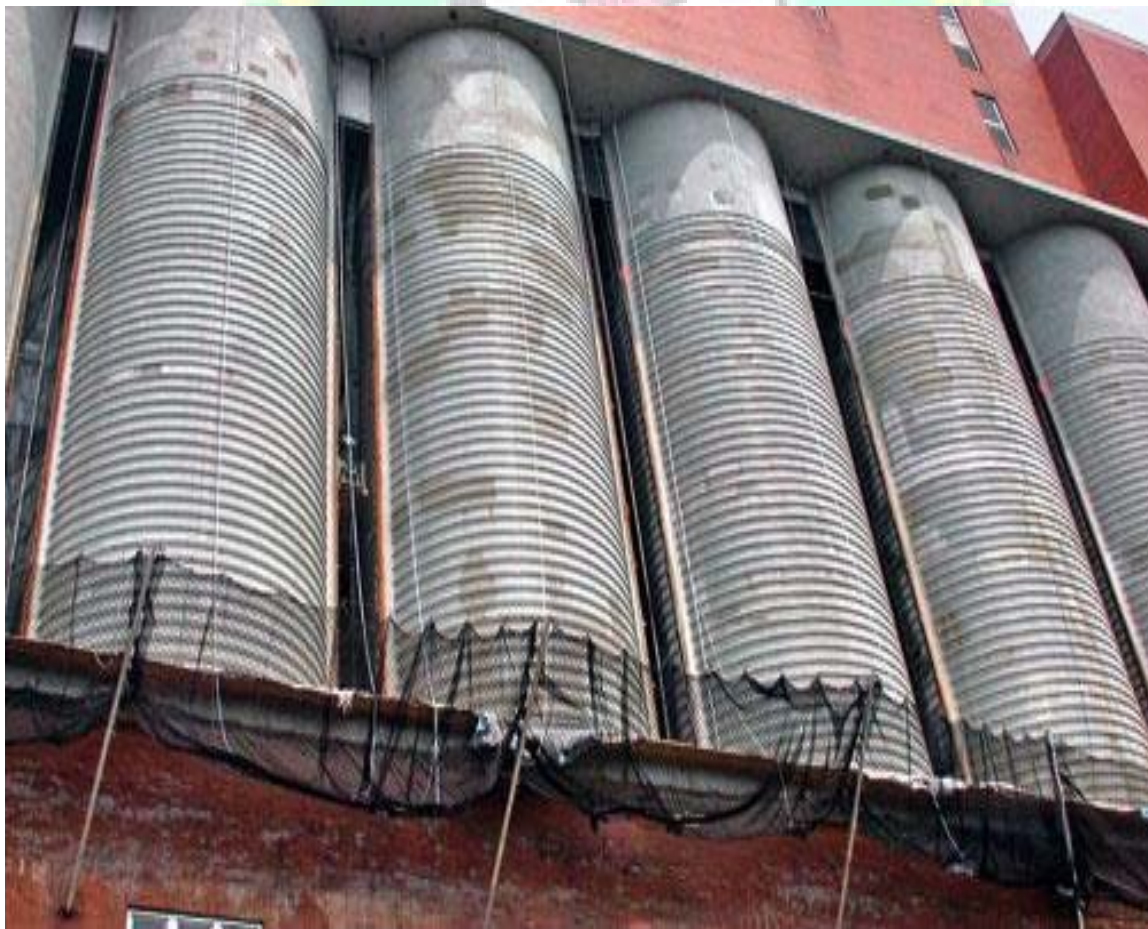
Figure: External prestressing in circular tanks
