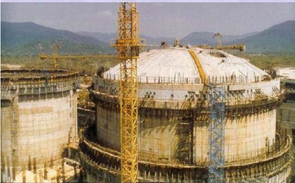
Figure: pre stressing of circular tank
